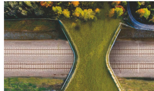
Bridges, culverts or so-called ecoducts are proposed for the surface route. Their purpose is to allow easy passage for all animals.
